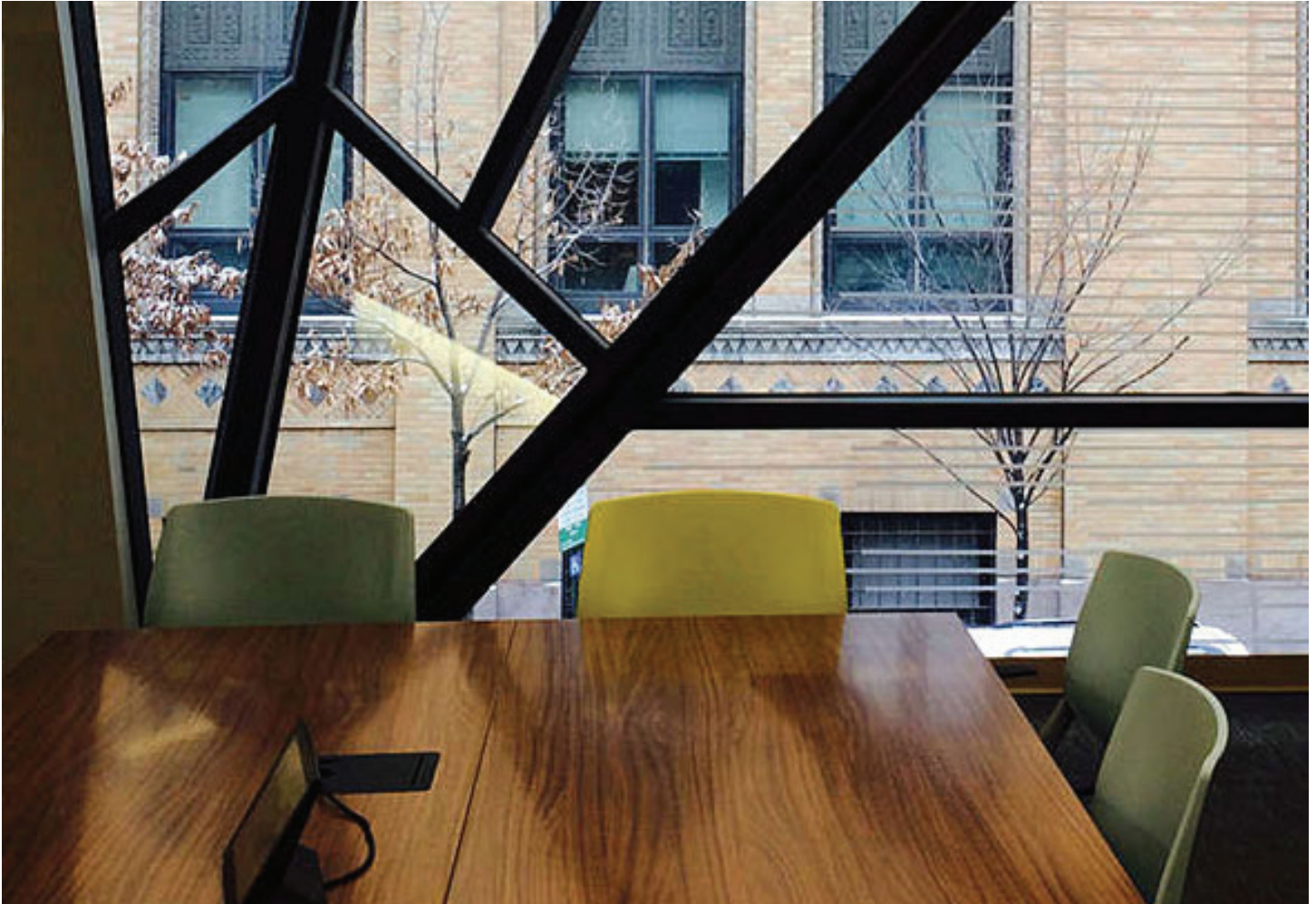
A view of the second-floor interior of the 10th Street innovation hub. As the glass facade of the Jefferson Accelerator Zone project begins to fan out, it forms an off-kilter crystal protrusion that extends just three feet over the sidewalk - the legal limit.
